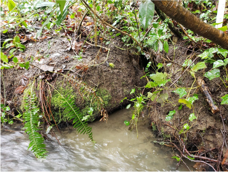
Photo 7. Stormwater conveyance channel confluence with Stream A.
