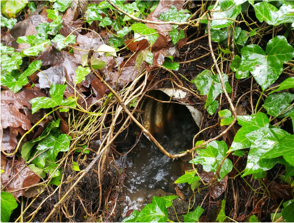
Photo 5. 12-inch stormwater pipe outlets to conveyance channel.
